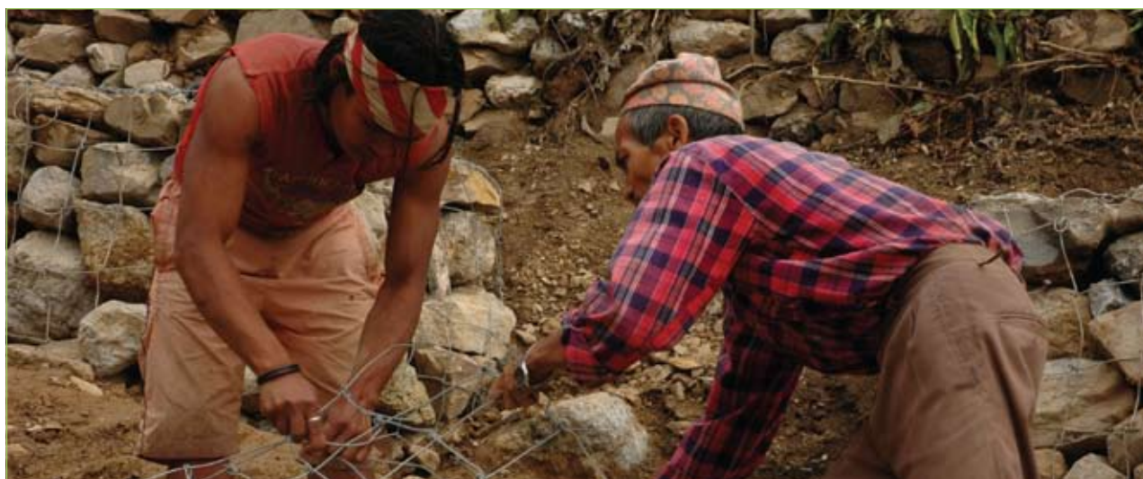
Construction of gabion to protect irrigation canal from flooding, Chitwan, Nepal
